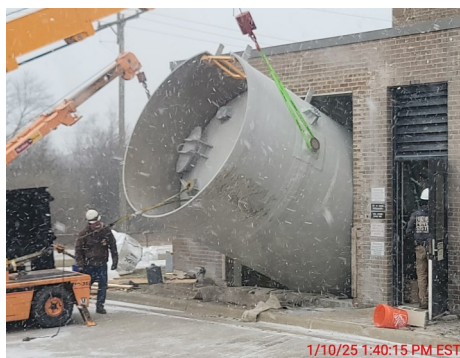
Pictured: Installation of a new chemical storage tank.
